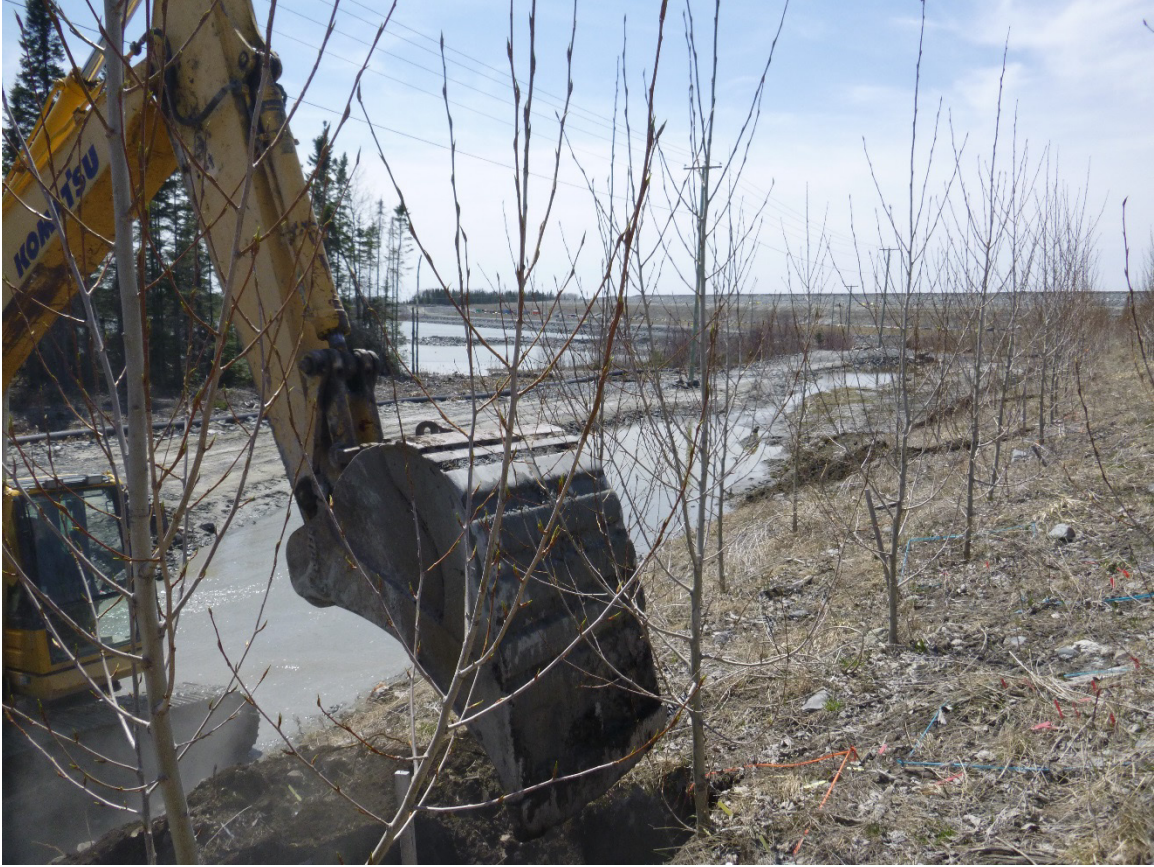
Figure 3: Trenches made with a mechanical shovel to determine the maximum rooting depth.
