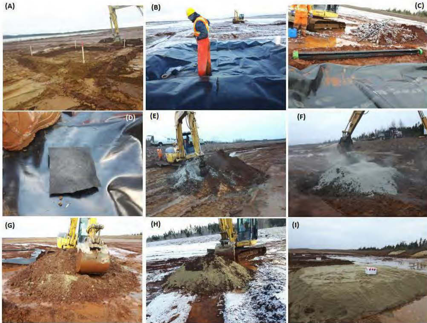
Figure 7.1 : Images showing field cells construction and amendments mixing with oxidized tailings (A, B, C and D : cells excavation, geomembrane and drains installation, E, F, G, H, I: amendments mixing with oxidized tailings)
