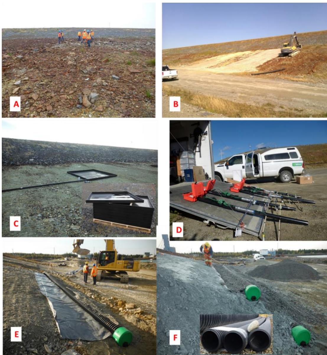
Figure 7.2. Photos illustrating construction of the inclined experimental cell.
