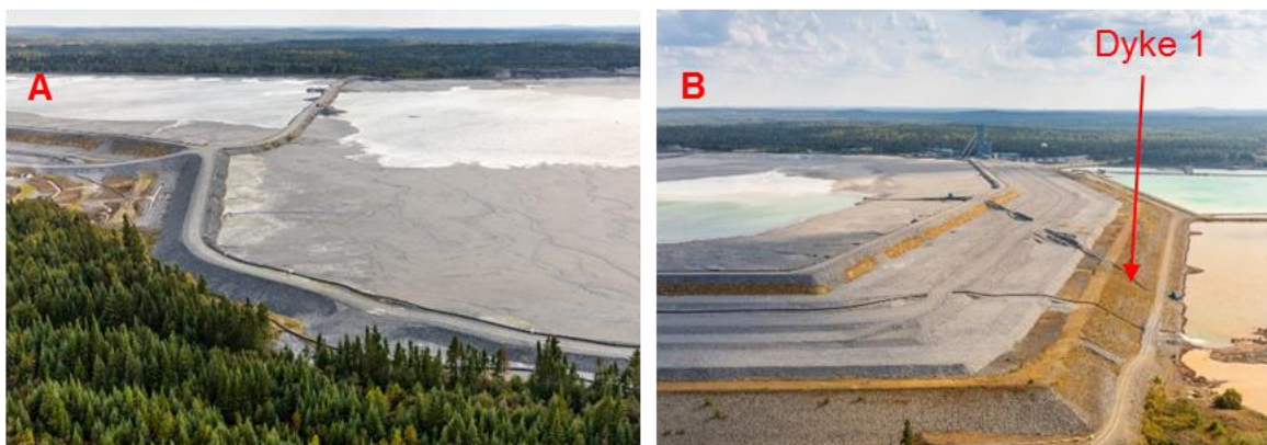
Figure 7.1 Acid generating LaRonde tailings storage facility.
