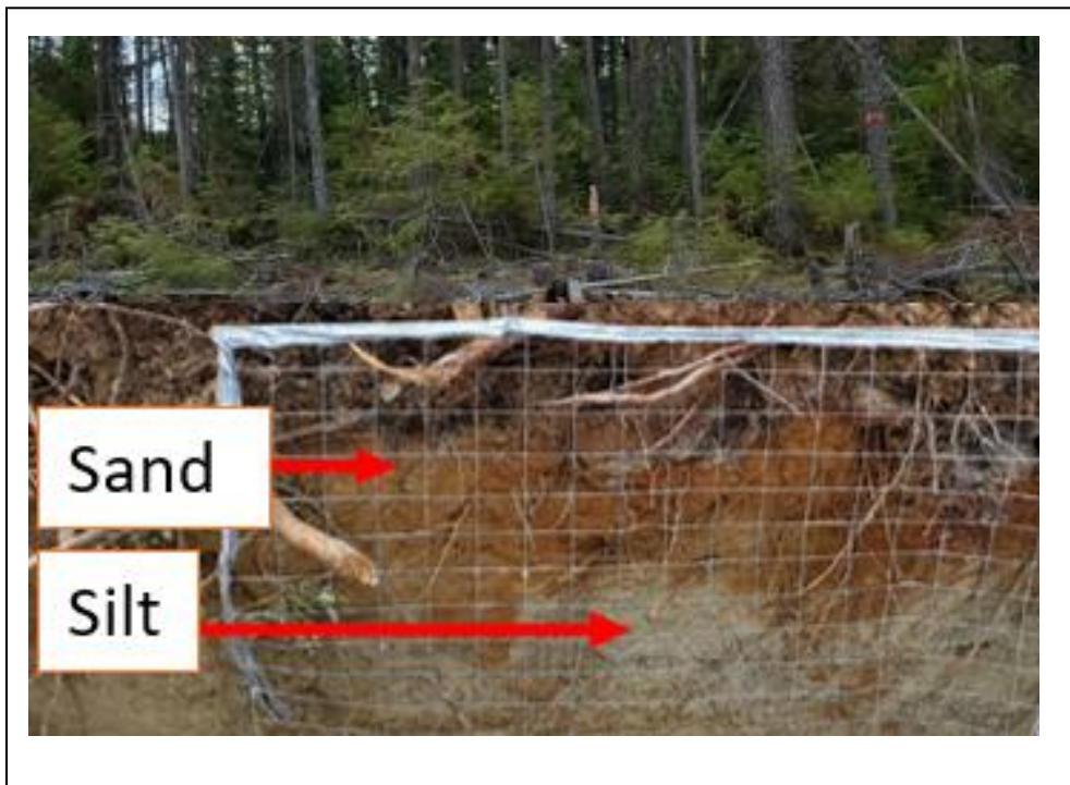
Figure E.1 The substrate profile of the selected site for the NA of a CCBE (composed of a sand layer above a silt layer) colonised by mature Pb vegetation (adapted from Cissé et al., 2022)
