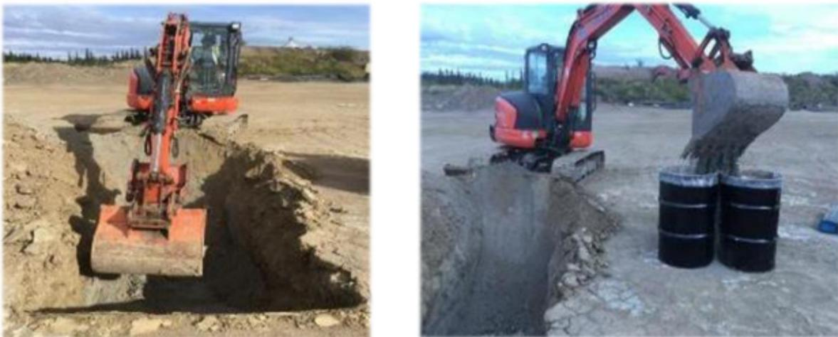
Figure 3.9 Excavation and sampling of the tailings at the Giant Mine tailings impoundment
