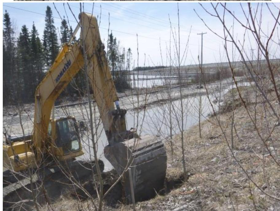
Figure 5.2 Trenches made with a mechanical shovel to observe the vertical profile of roots
