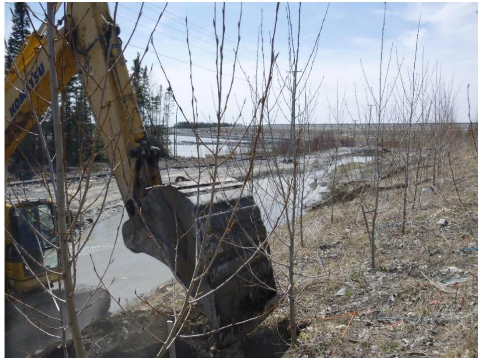
Figure 6.3 Trenches made with a mechanical shovel to determine the maximum rooting depth
